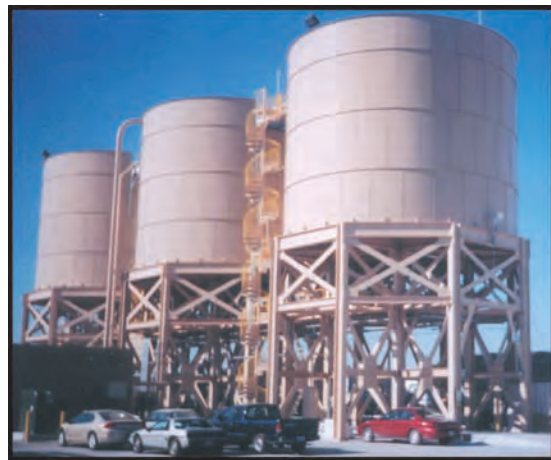
California Portland Cement - North Las Vegas, Nevada
